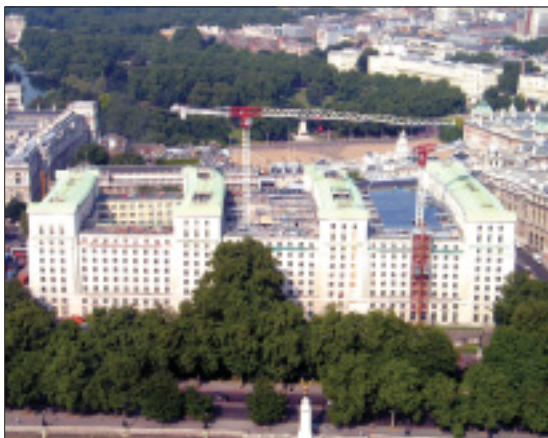
Construction work on MOD's Main Building is progressing ahead of schedule.
